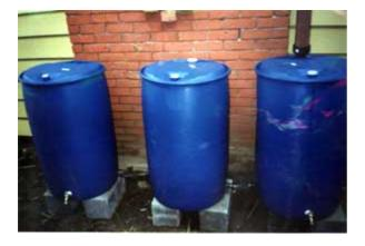
Step 5: The final product. You must attach an overflow line on the first barrel (the one on the far right in this picture). This must be placed near the top of the barrel and it should be attached to some form of hose or tube to discharge any overflow. Please note that you must remove one of the two bung fittings
