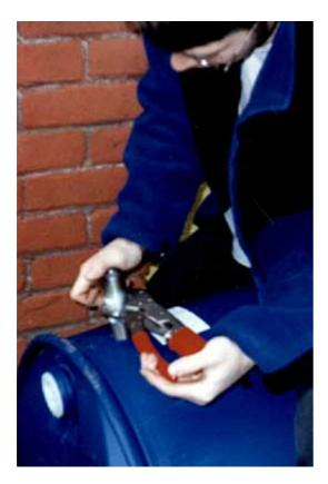
Step 2: Place plumbers goop on a 3/4 inch nipple. Using a 3/4 inch galvanized metal nipple and some locking pliers, thread nipple into the barrel. the hole for
