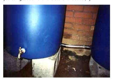
Step 4: If you are adding more barrels do this now. Attach a garden hose Y fitting on the 3/4 inch nipples. Position the barrels on top of the concrete blocks and cut the right length of garden hose to connect the barrels (with male fittings attached to both ends).
